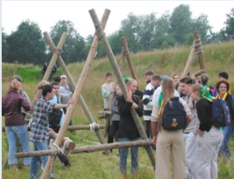
Building the amphitheater
